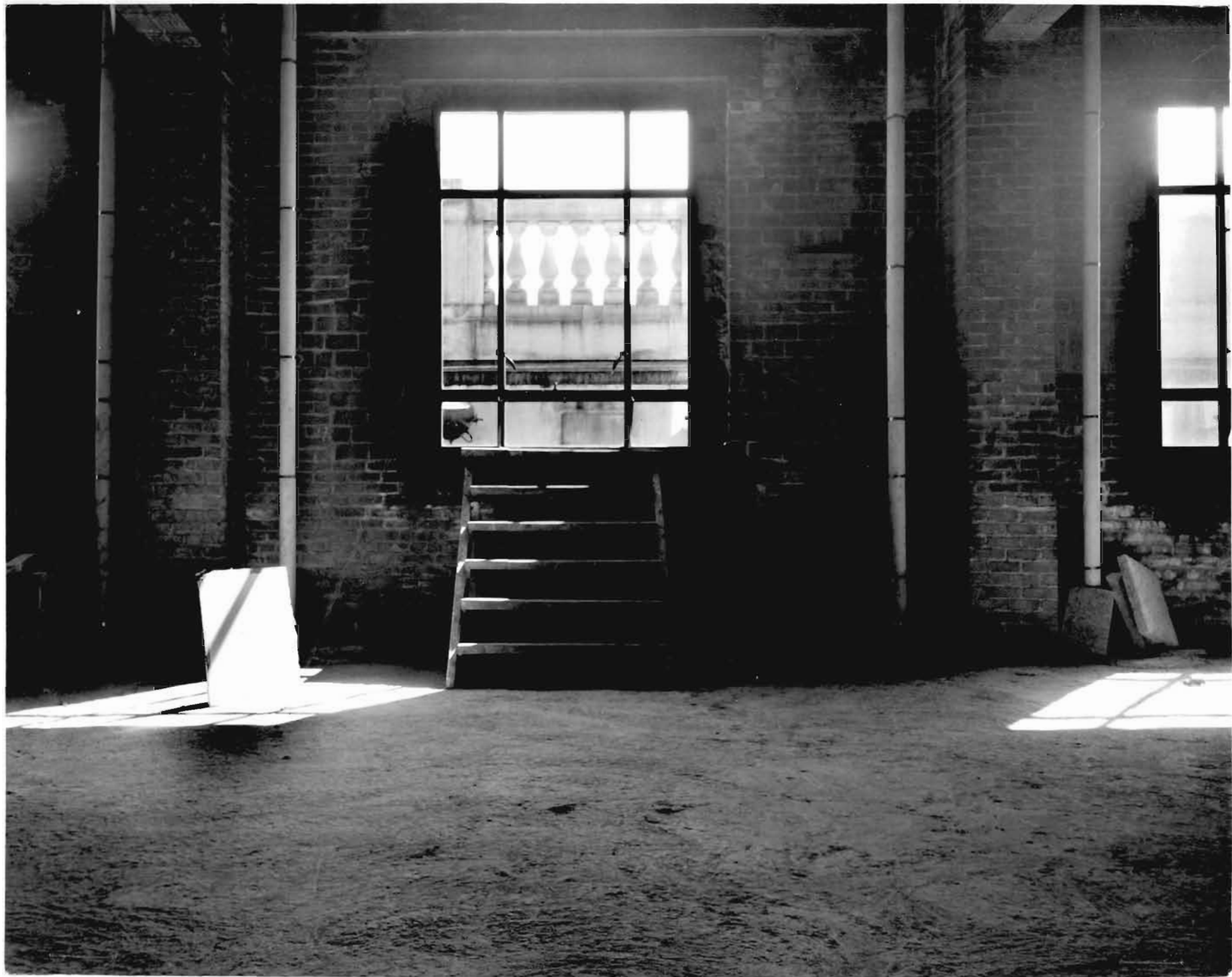
4. VIEW OF WINDOW ON SOUTH SIDE OF 20TH FLOOR SHOWING POSITION OF BALUSTRADE OUTSIDE OF WINDOW
