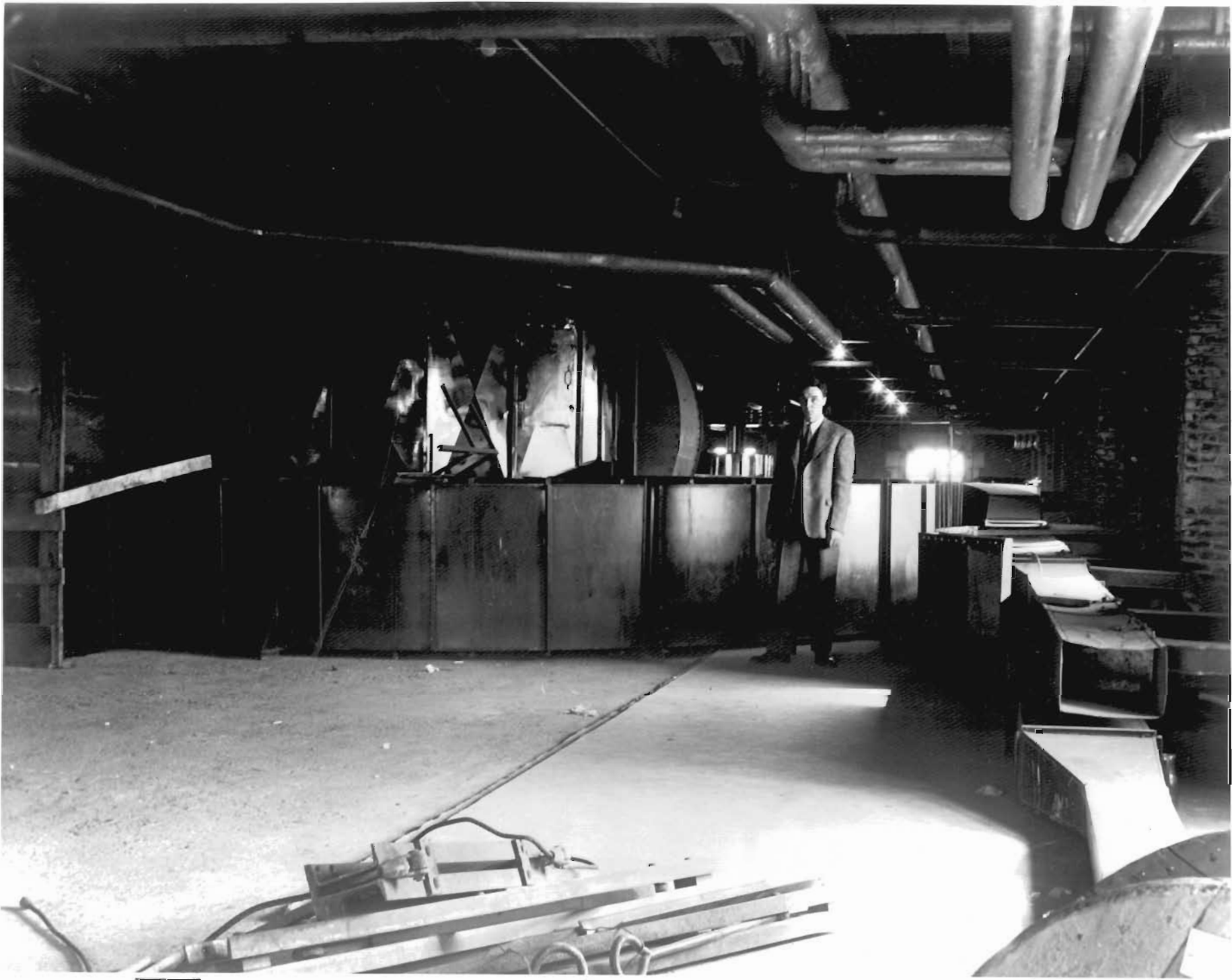
7. 24TH FLOOR (PIPE & DUCT FLOOR) SUN LIFE BUILDING, MONTREAL.
